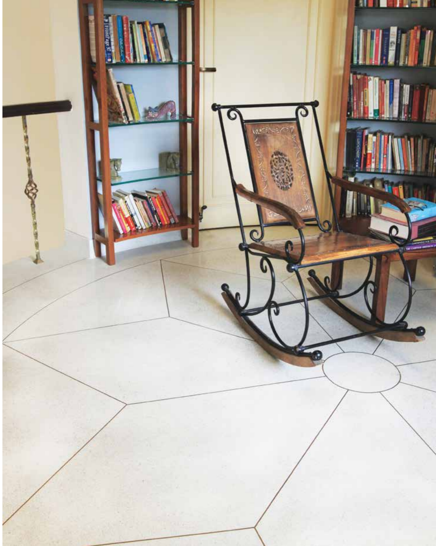
Cast in situ Terrazzo floor done using Brass strips and Cream Italian chips on White base, New Delhi. Interiors: Nikhil Sehgal.
