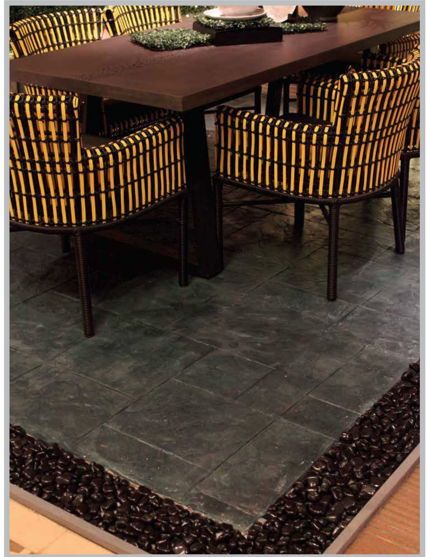
Thin Finish Stamped Overlay micro cement floor.
