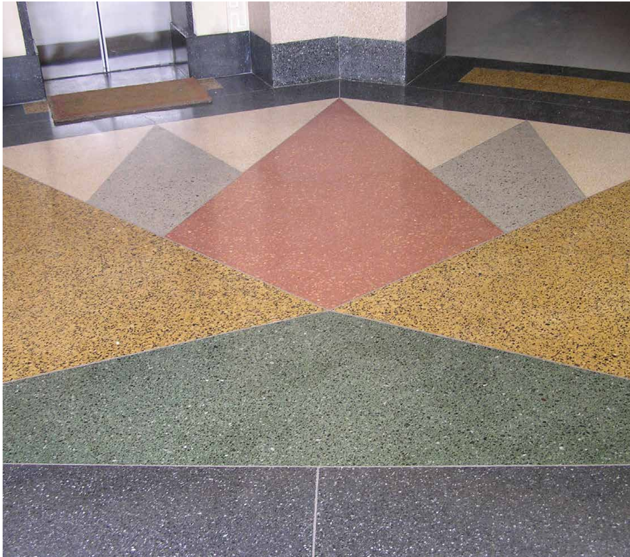
Cast in Situ restored at Kamal Mahal, Mumbai. Interiors: H Carnac
