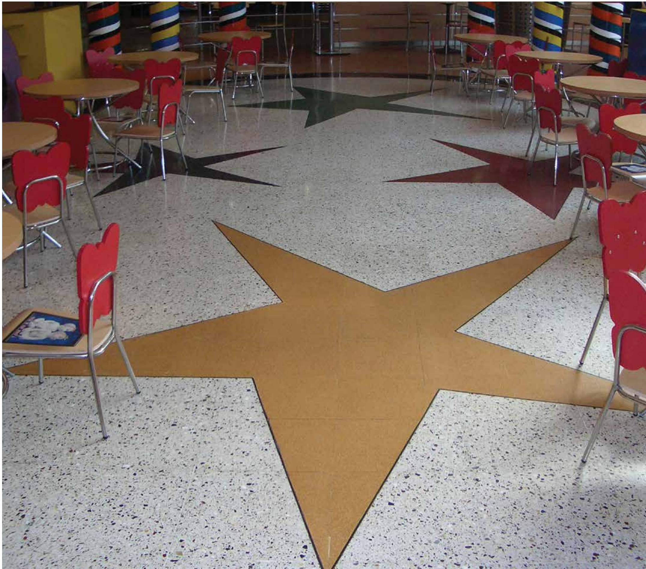
Cast in Situ Premium Terrazzo in Jaisalmer Yellow, Dark Green, Deep Red with plain designer stars at Inorbit Mall, Malad.
