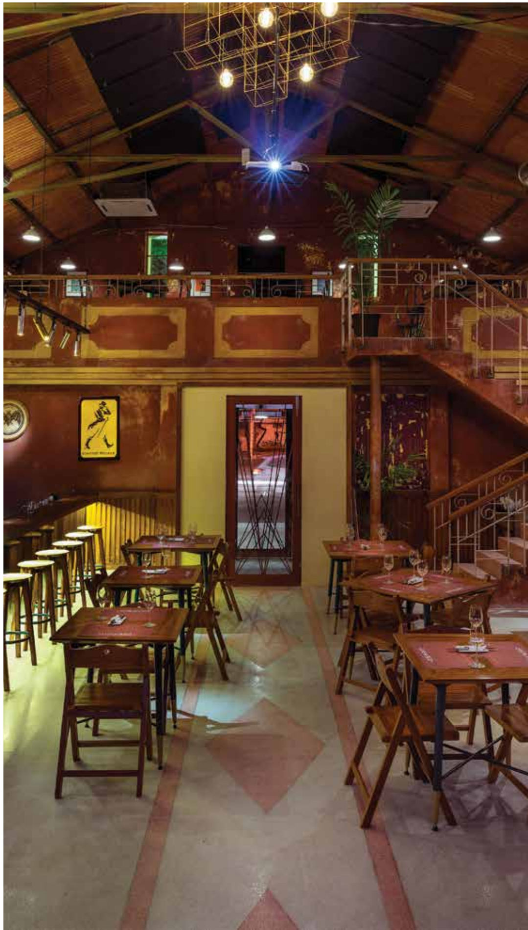
Cast in situ Terrazzo flooring in shades of Teracotta red and Silver grey at a pub, Showbar in Candolim, Goa. Interiors: Raya Shankwalker Architects.
