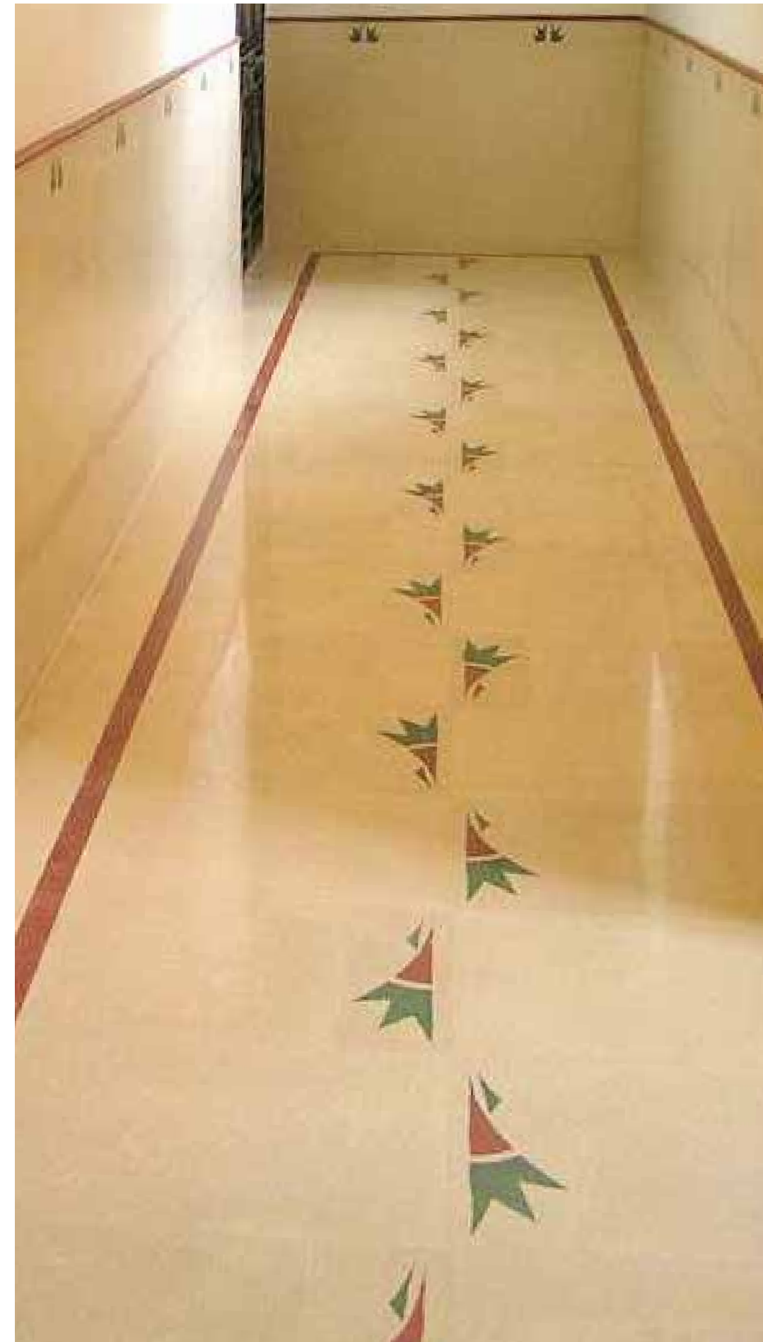
Sicilia and Cream Italian slabs used at the Les Palmes lift lobby with a custom motif. Interiors: H Carnac.
