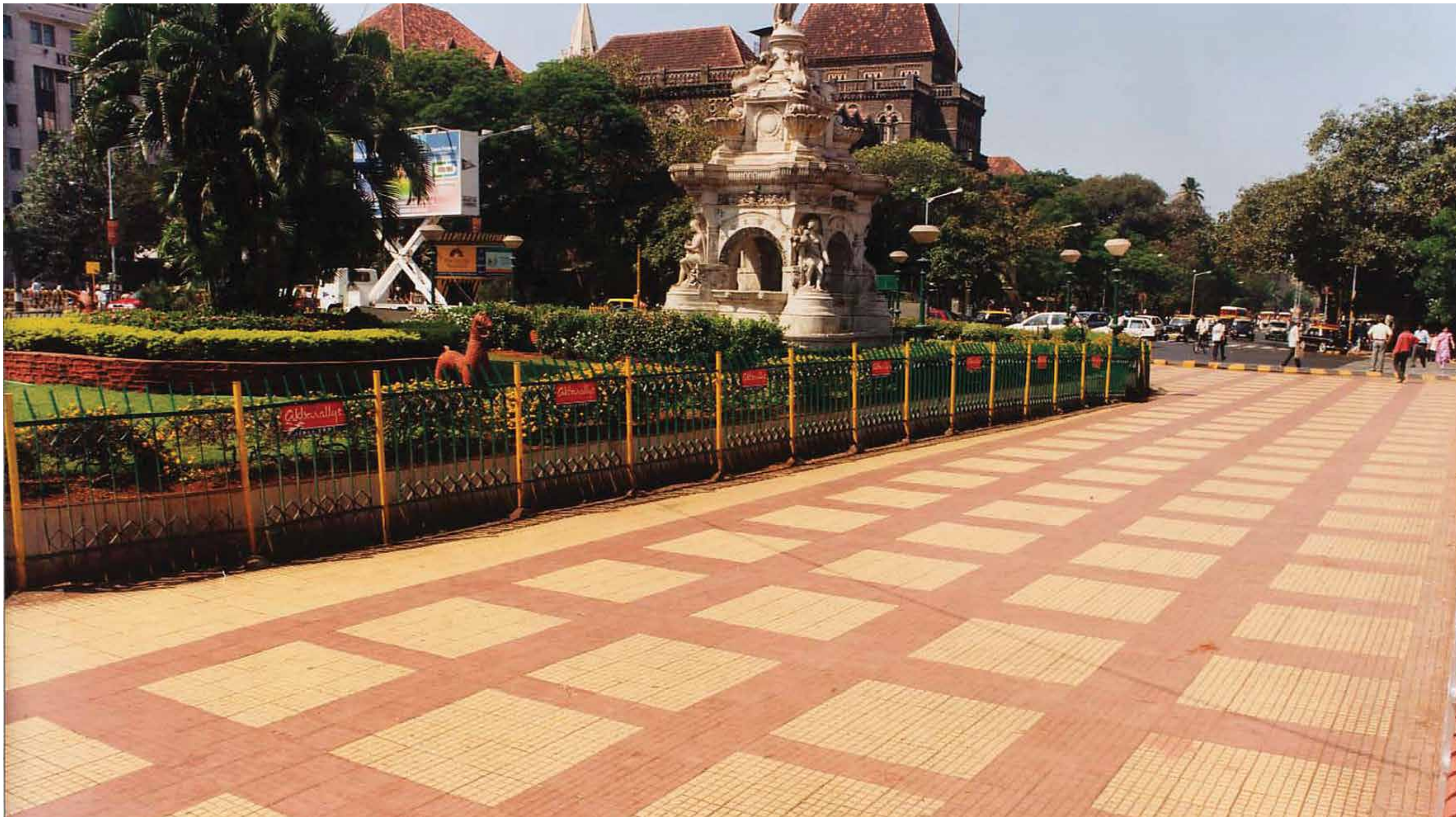
Flora Fountain floored with Stilan® Non Slip tiles.
