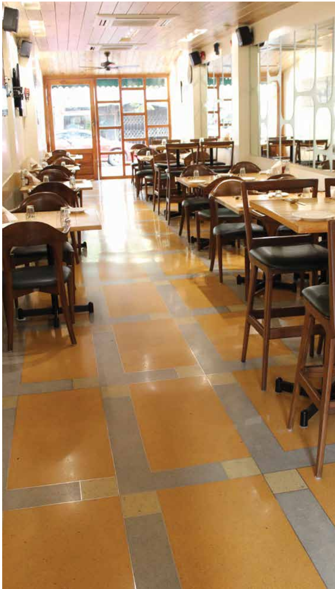
Cast in Situ Terrazzo tiles in Sunshine Yellow, Buttercup Yellow and Grey colours at Eddies Bistro, Mumbai. Interiors: Studio Osmosis
