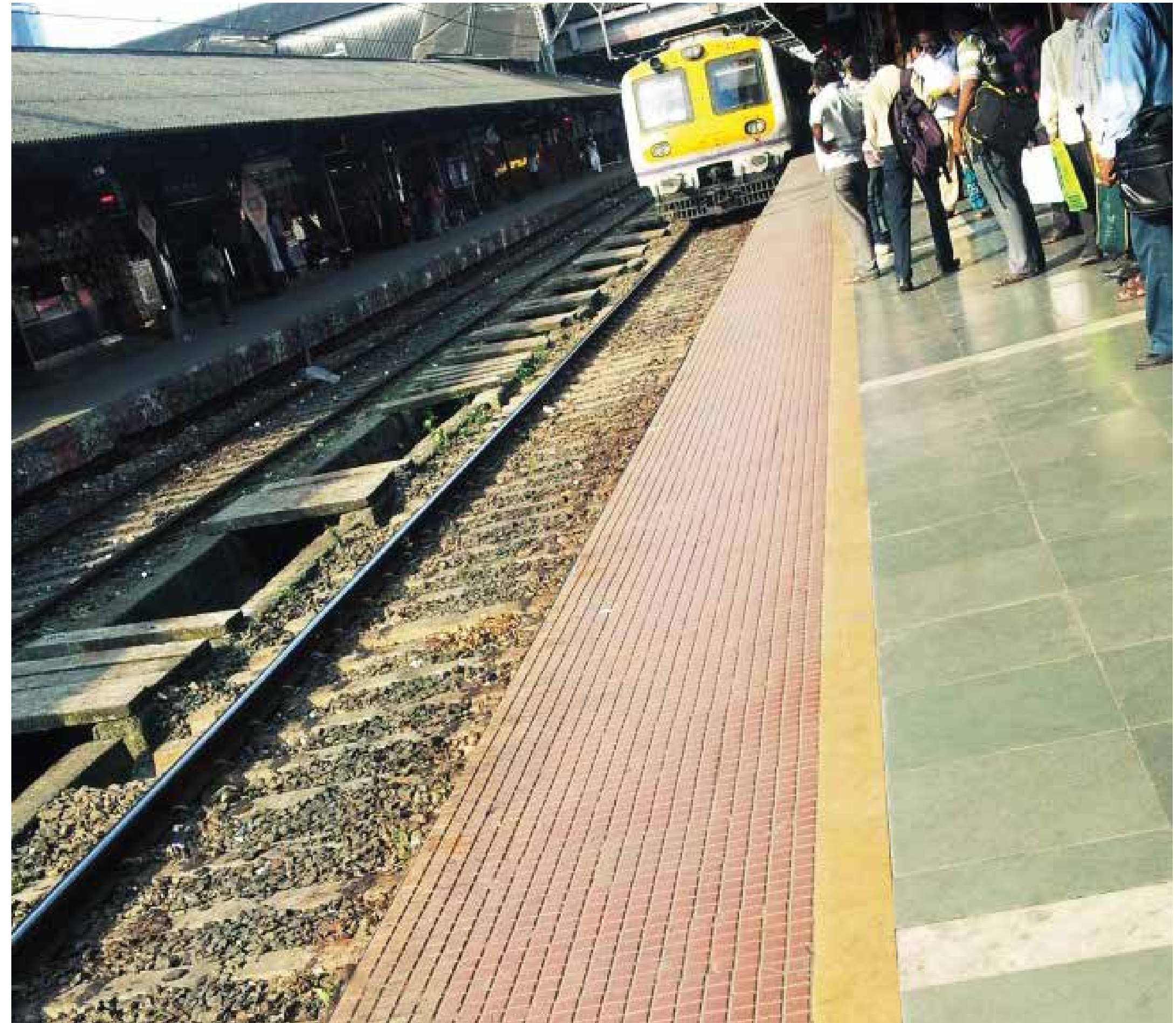
Railway platforms have borders of Stilan® Non Slip tiles.
