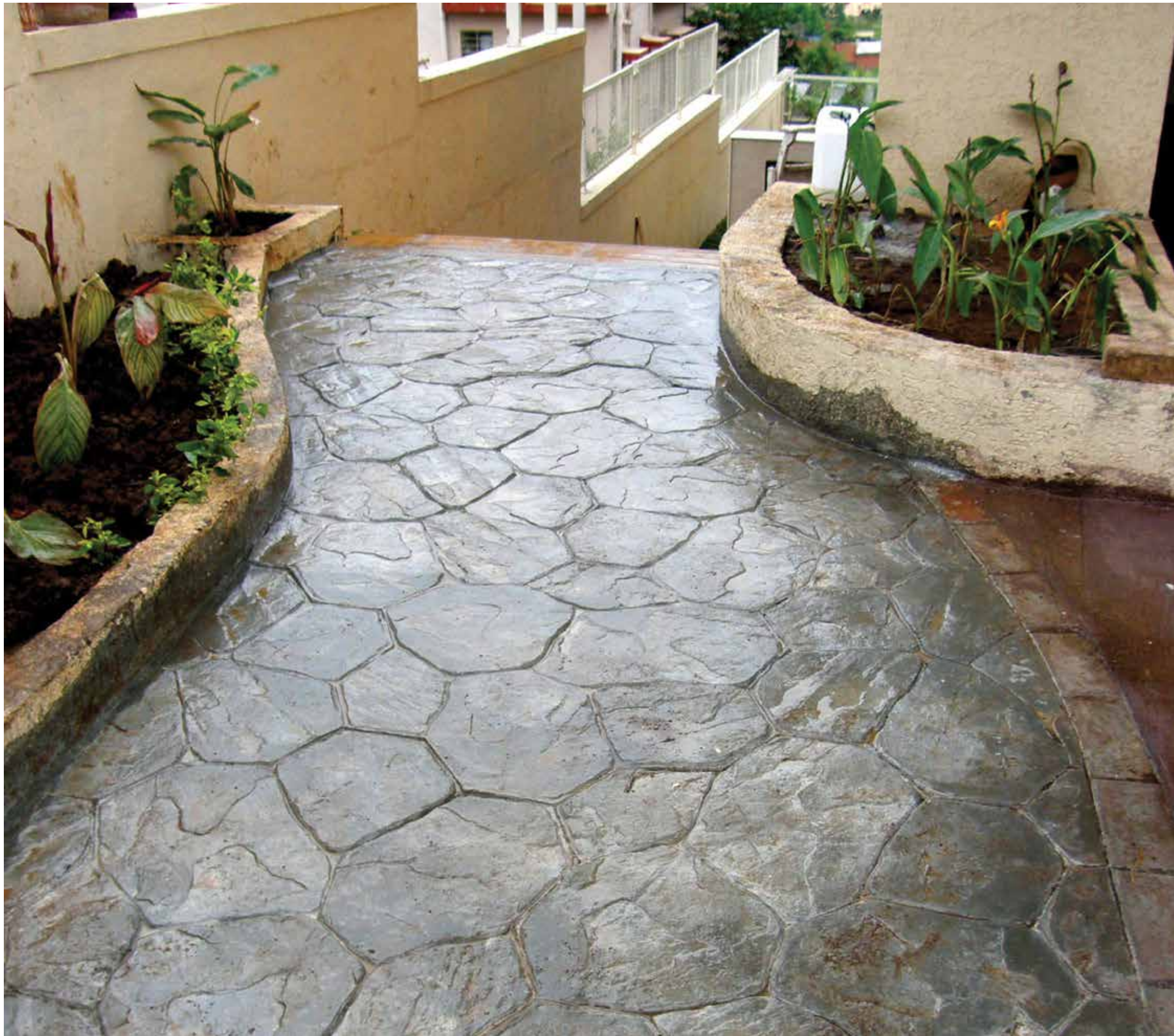
Random stone Terra Natura™ in slate grey colour used in a walkway at a house in Pune.
