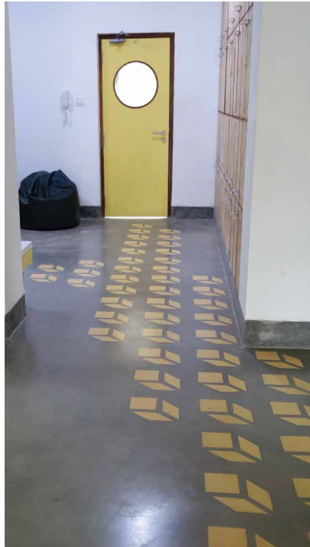
Cast in Situ IPS tiles in Buttercup Yellow and Grey colours at IT firm Tamera Projects, Bengaluru. Architect: Atelier Associate.
