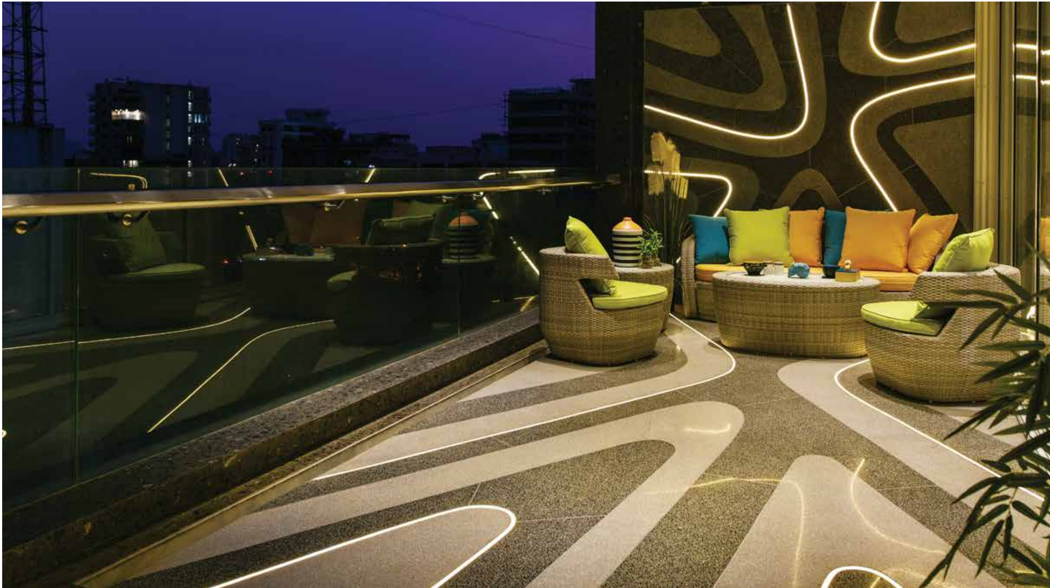
Cast In Situ Terrazzo floor and wall in Grey and Light Silver Grey colours. Interiors: Studio Osmosis
