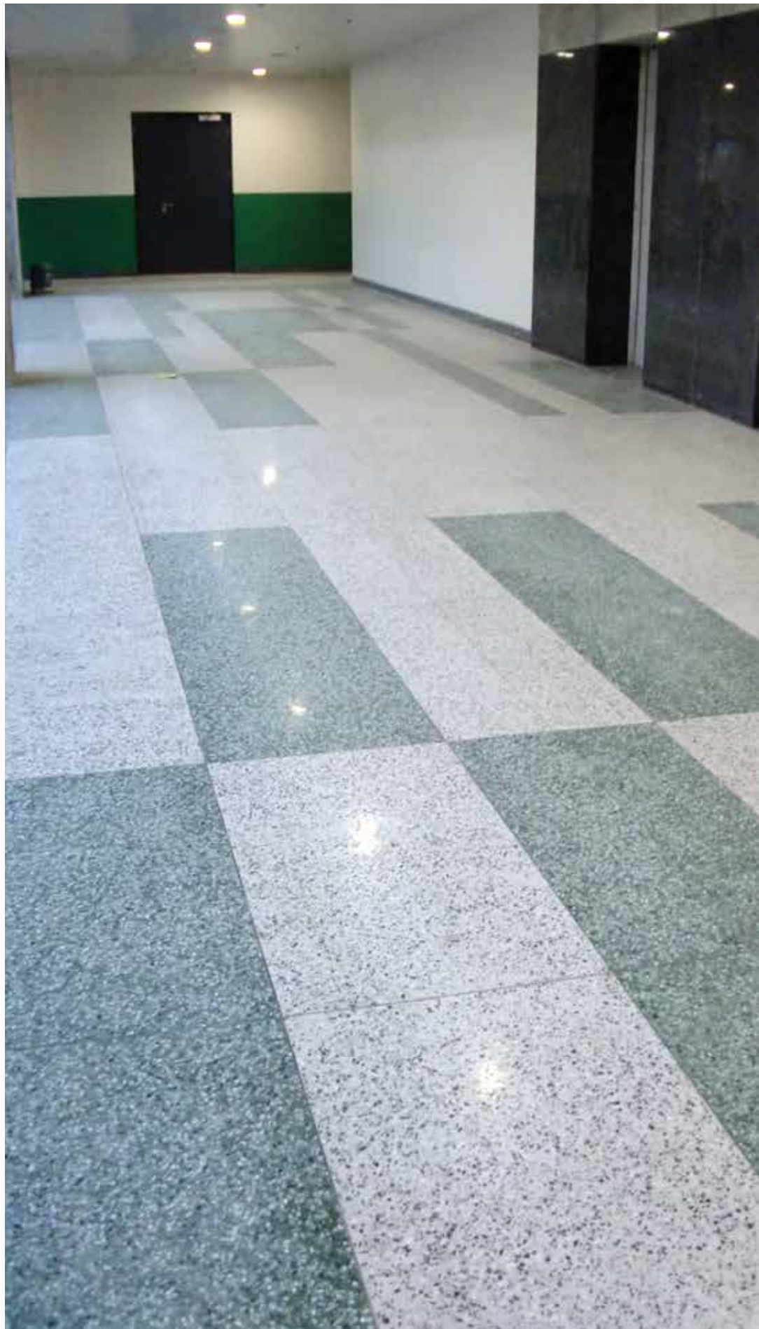
Cast in Situ Terrazzo in Grey and White colours at Tata Consultancy Services offices, Pune.
